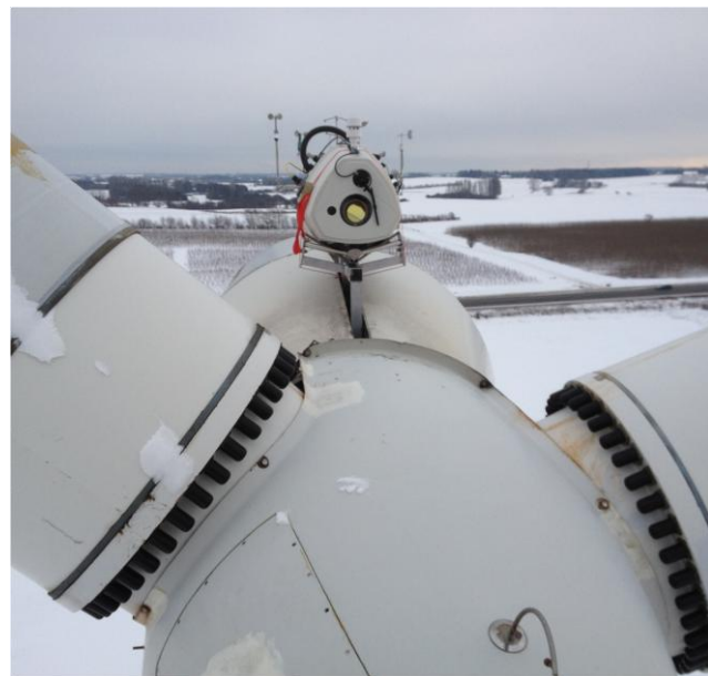
Figure 1: ZephIR DM installed on nacelle of turbine at DTU Risø Campus
