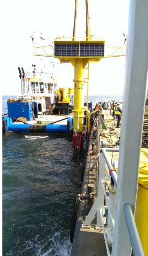
Figure 3: Installation of the low-motion spar buoy.
